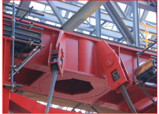
Figure 10. The strand connection with the starter beams.
