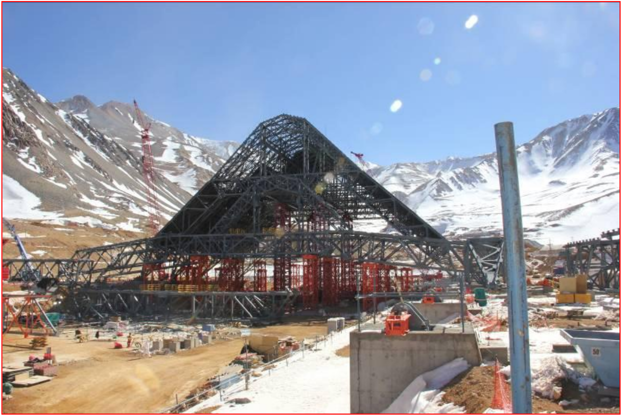
Figure 15. The jacked up roof from the opposite direction.
