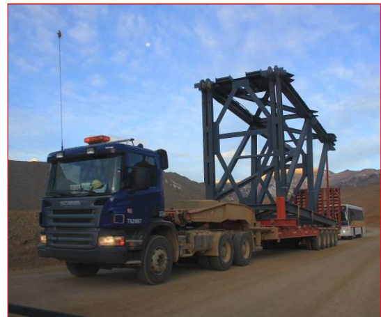
Figure 3. Complete truss sections are transported to the mine
