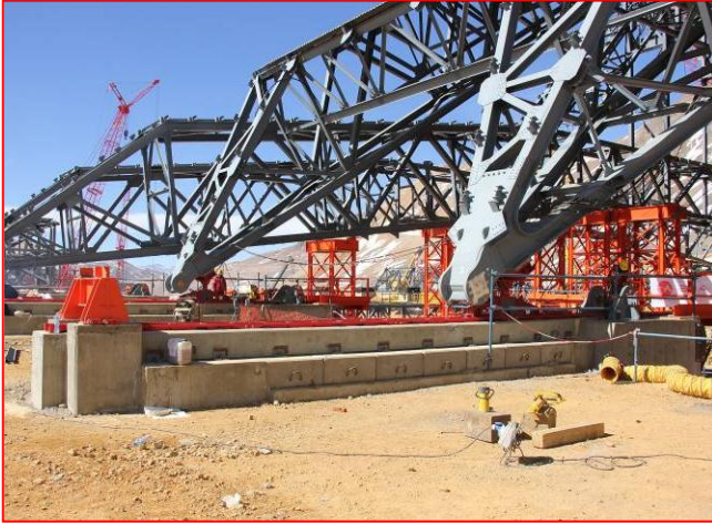
Figure 9. A side view of the hydraulic skid, at the skid lane in action.
