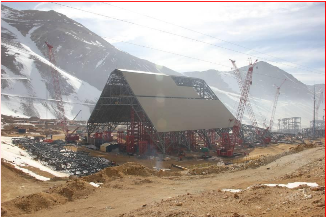
Figure 16. The stockpile building from a distance in final position.
