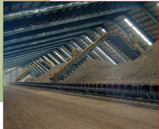
Figure 2. Example of a stockpile building
