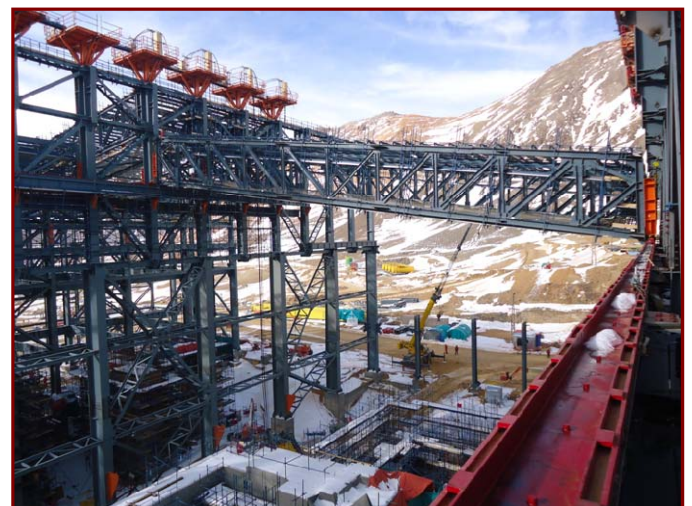
Picture 3. Frame number 2, skidded to its lifting position.
