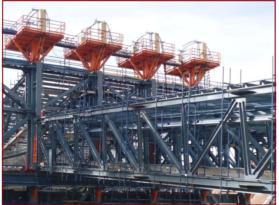
Picture 5. Strandjack in consoles, anchorages in frame number 2.
