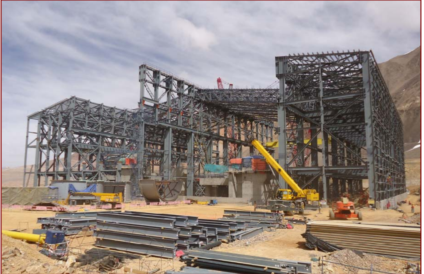
Picture 10. Molienda Building with its 4 central sections in their final position.
