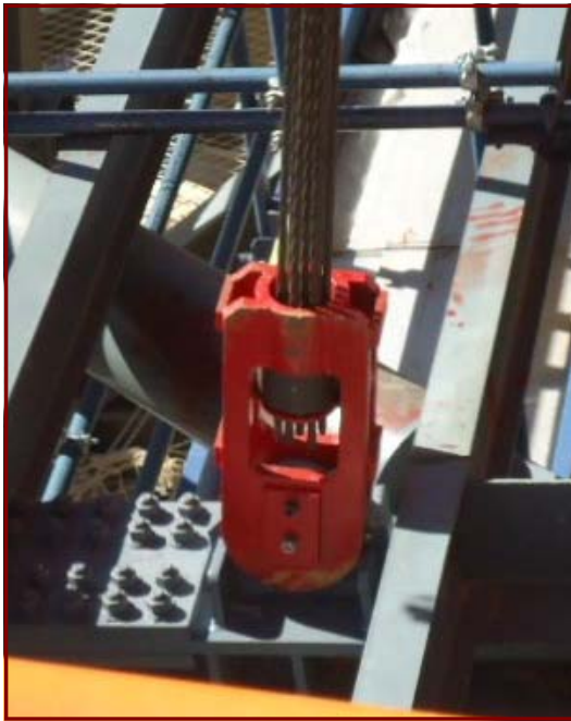
Picture 4. Anchorage and strands connected to the lifting lug.
