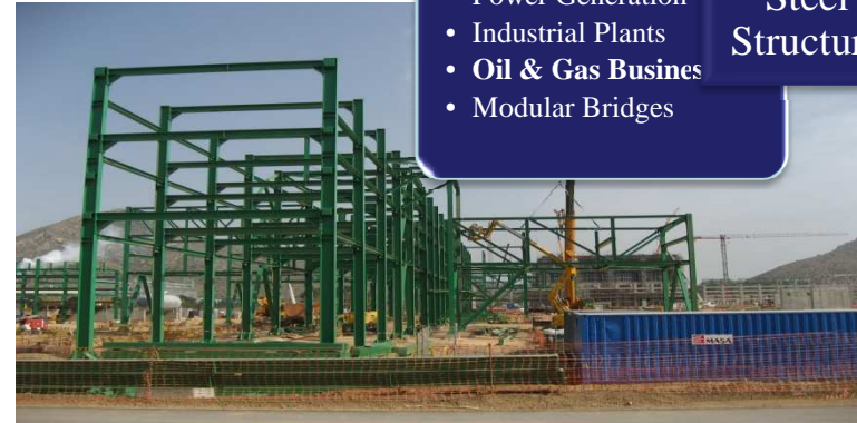
Client Repsol 2.011 Project Pipe Racks
