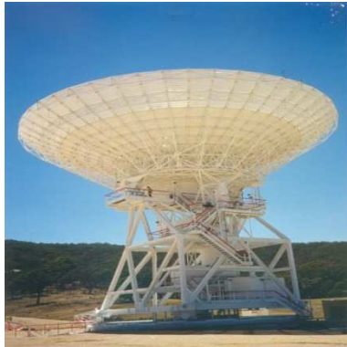
Client Deep space 1996 Location Australia Weight 400 mT (34m Diam)
