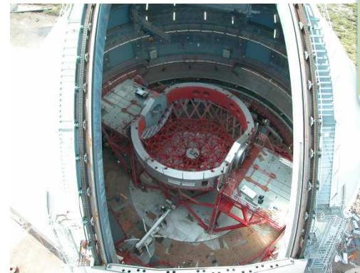
Client Telescope Erection on site Location Hawaii Weight 550 mT
