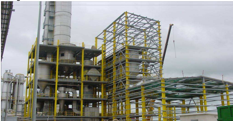
Client Fydsa, 2005 Location Spain (Almussafes) Weight 825mT
