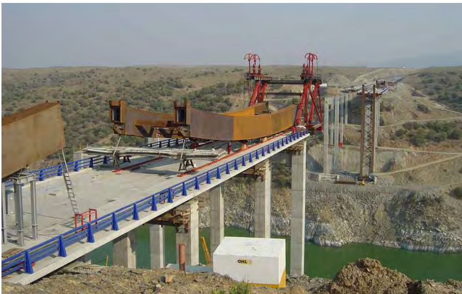
Skidding lower arch section
