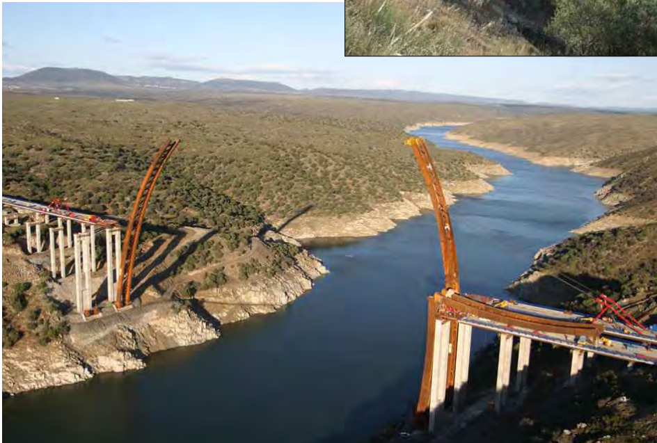
Skidding lower arch section
