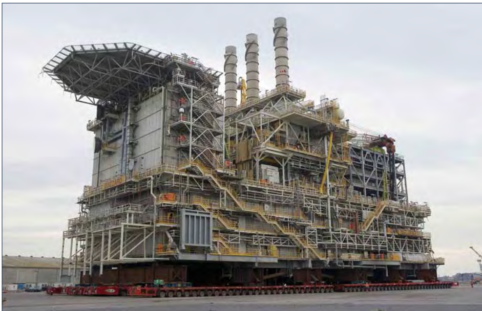
All axles controlled by single operator
