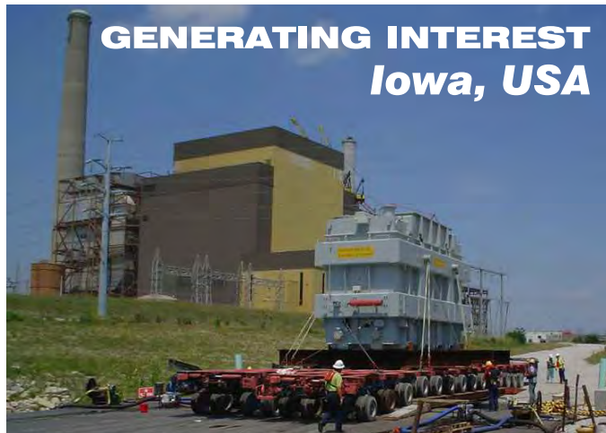
Transformer delivered to site
