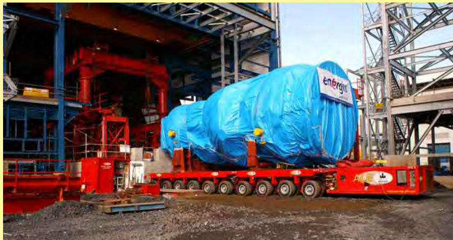
Above: Transport using SPMT
