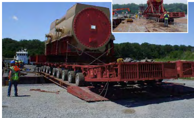
(Below and right): Off-loading generator and turbine from barge
