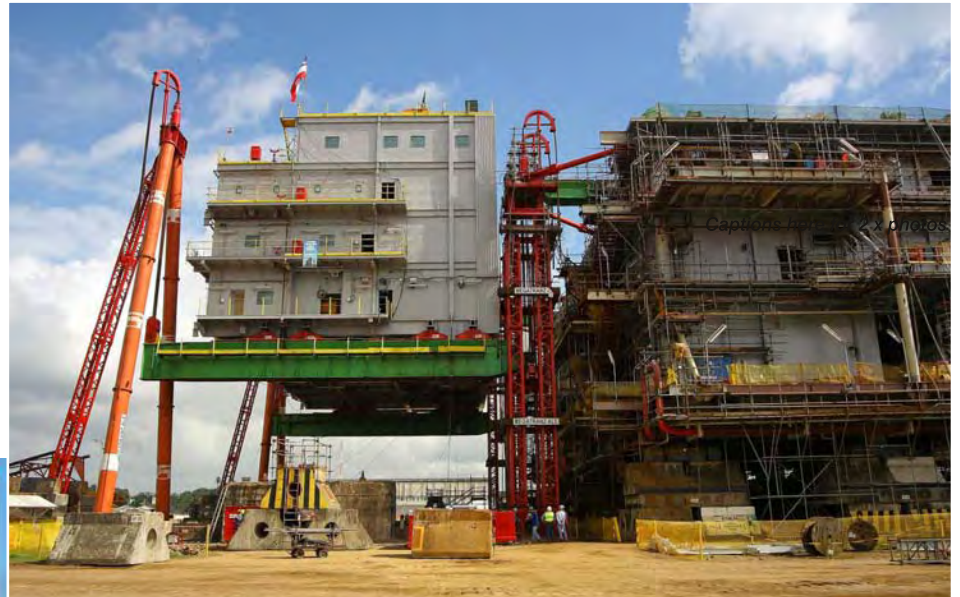
LQ Module lifted 25 metres
