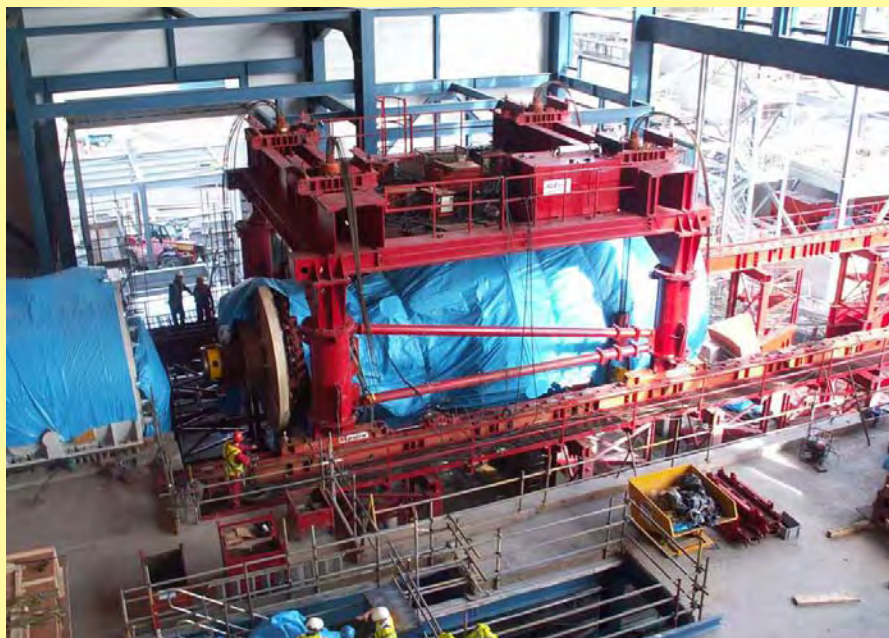
Below: Installation of Gas Turbine
