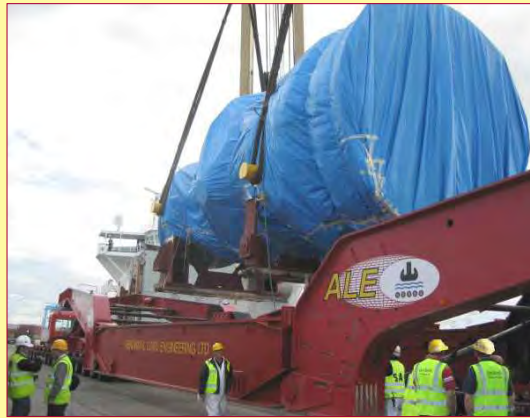
Gas Turbine lowered into Girder Frame
