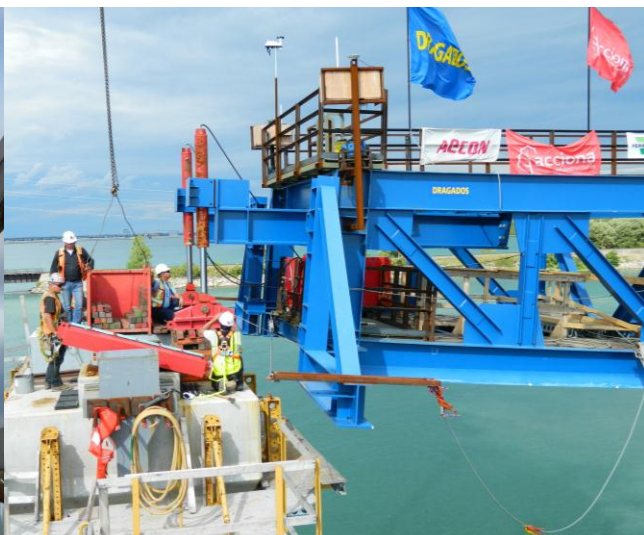
System to compensate the deflection at front section
