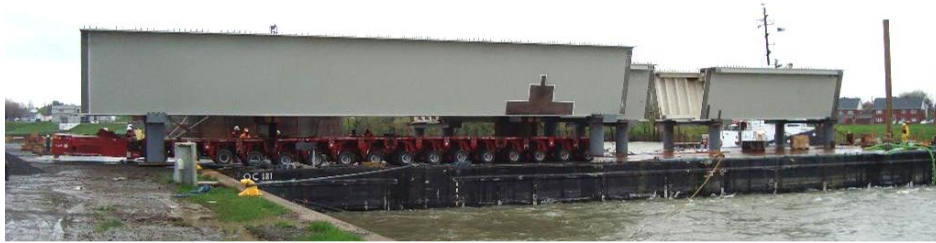
Load in / load out to the barge
